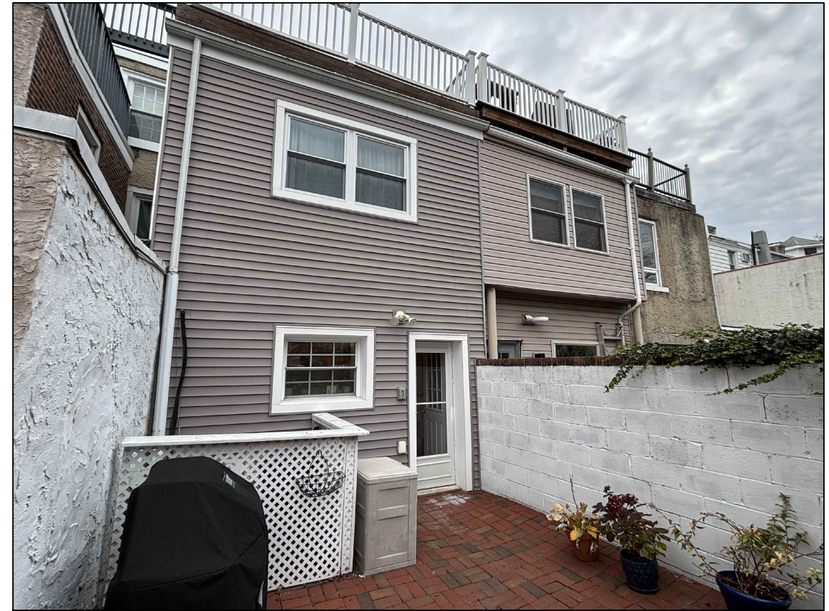
REAR FACADE LOOKING NORTHEAST
