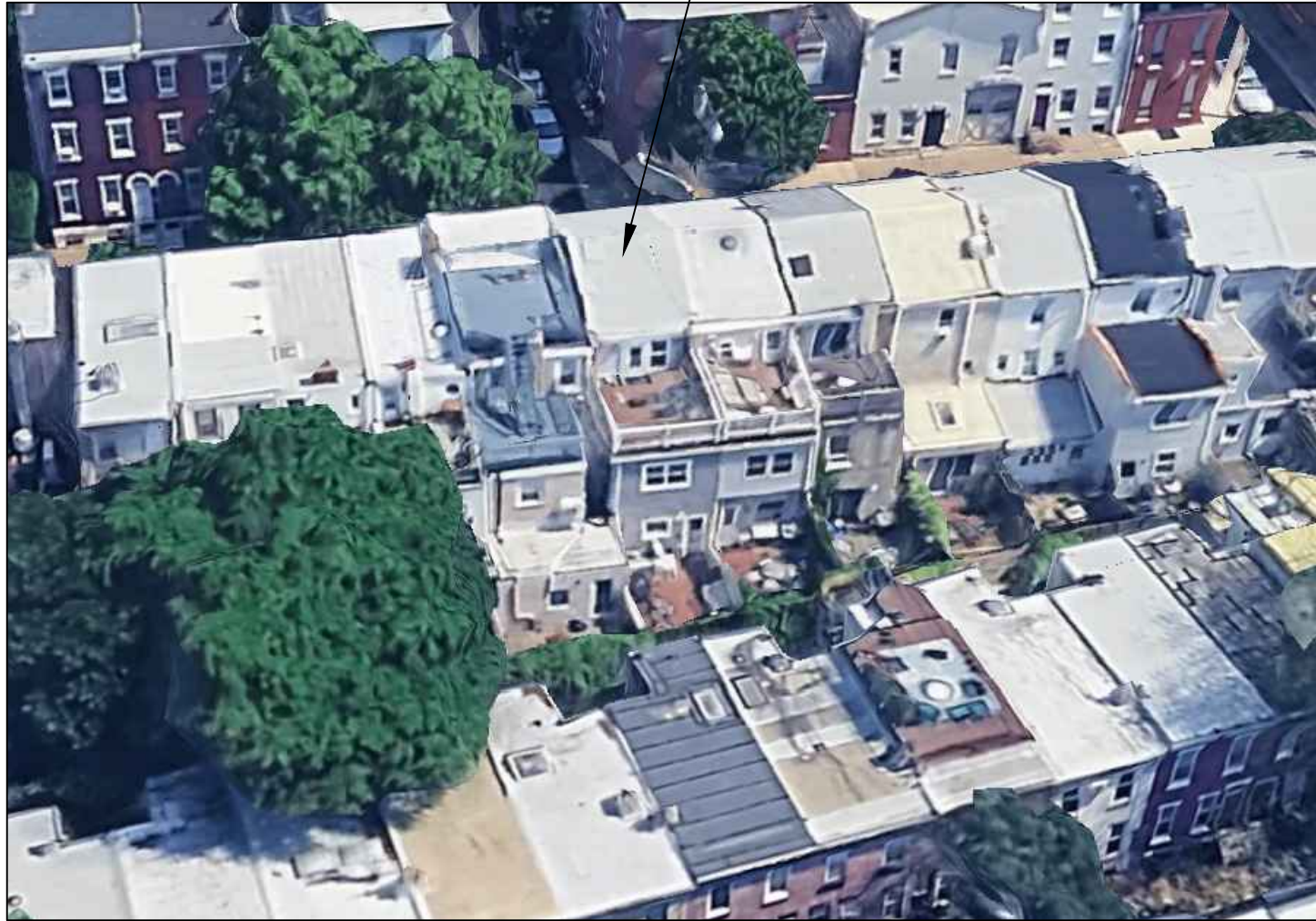
AERIAL VIEW LOOKING NORTH
