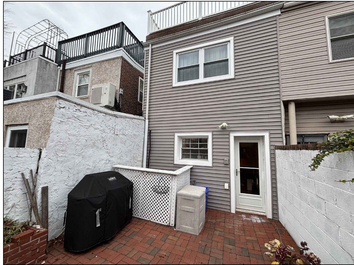
REAR FACADE LOOKING NORTHWEST
